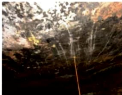
Fig: Joints exposed in the sandstone roof
