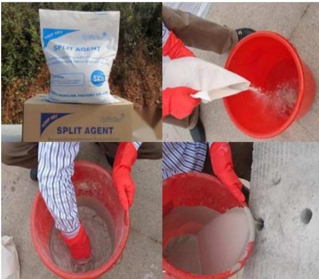
Figure: Mixing and Pouring of Expansive mortar (Crack Powder)
