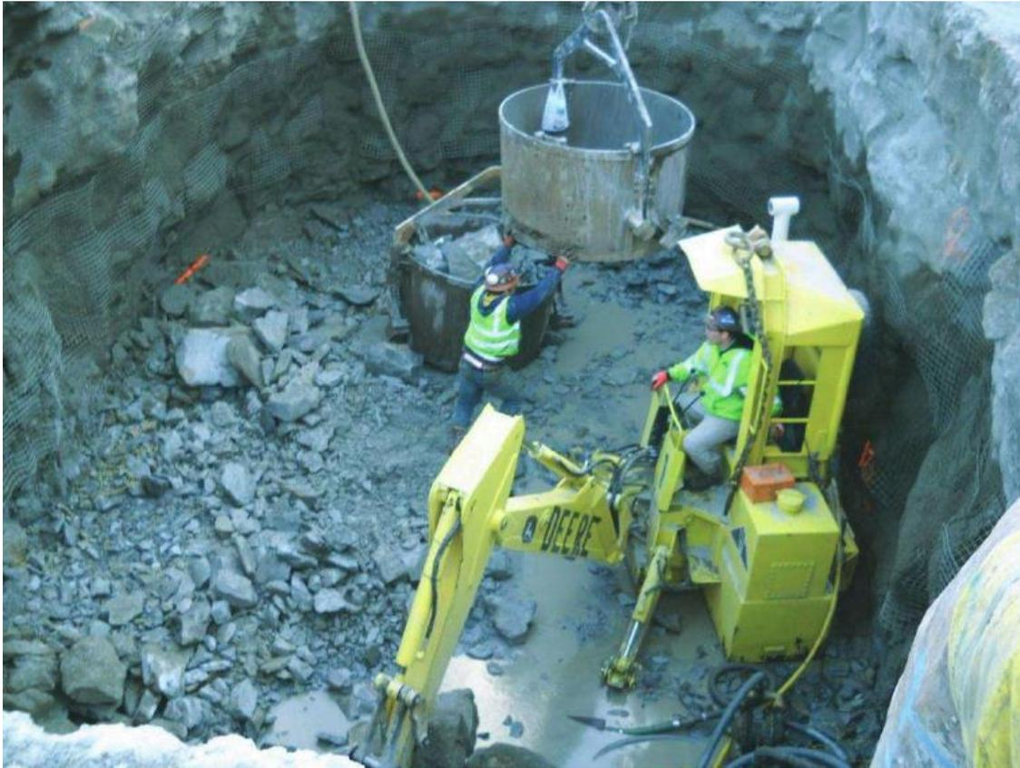
Fig – Operation of Mucking
